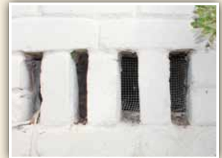
Check for loose mesh in foundation vents.
