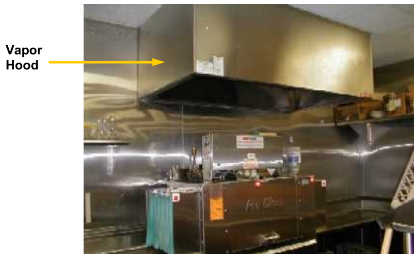
Figure 13. Type II Hood Over Dishwash Machine
