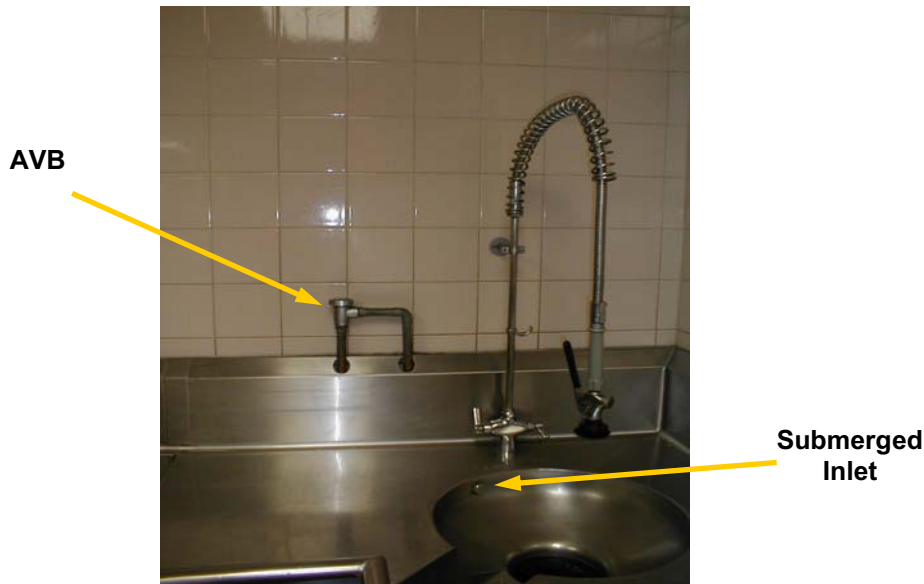
Figure 7. Vacuum Breaker with Submerged Inlet
